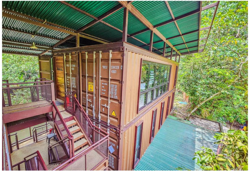
The space between the roof and the top of the containers is deliberately left open, so that the hot air that accumulates in this space from the sun, can disperse with ease, especially when it is a windy day.
