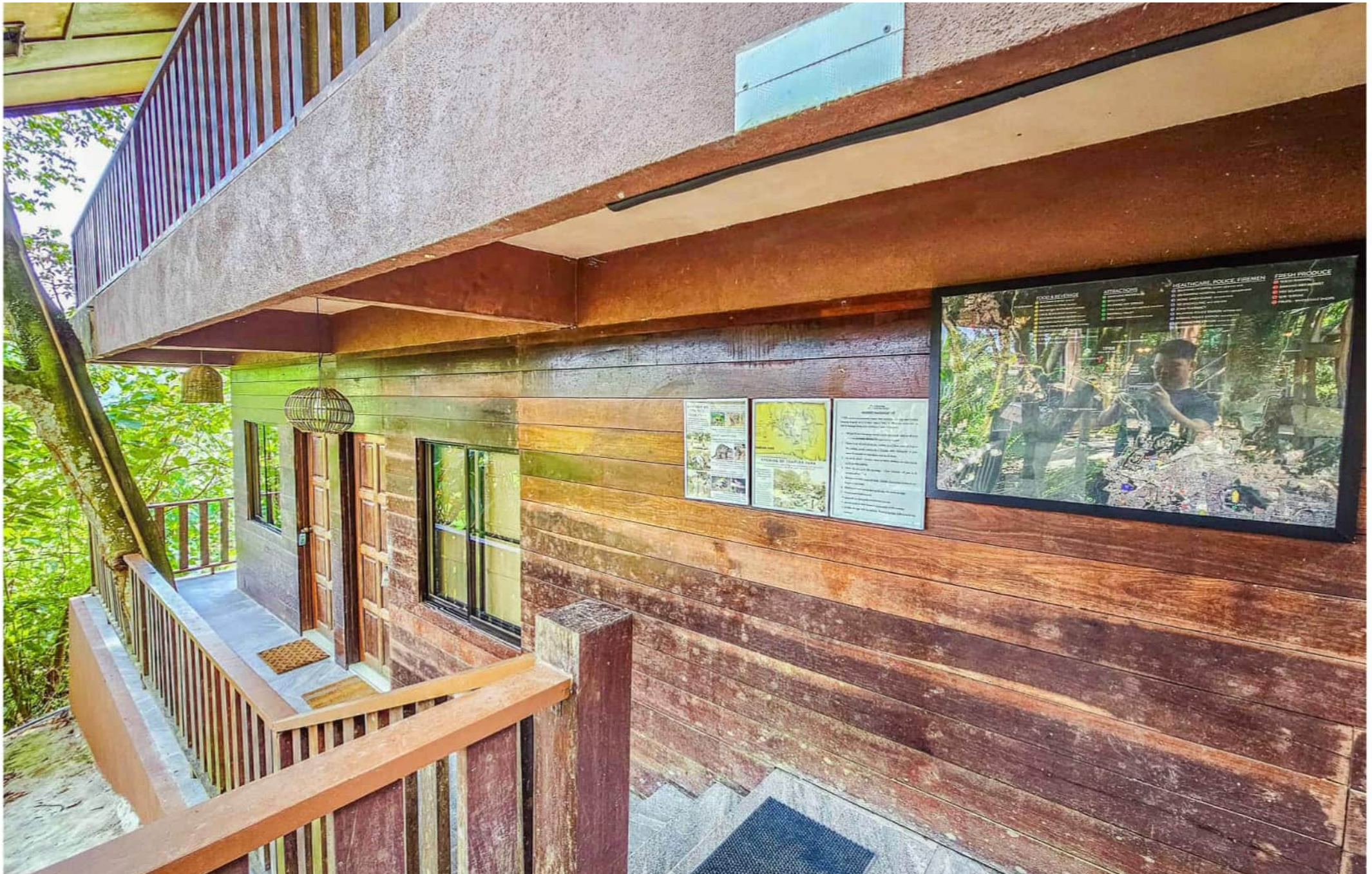
All bedrooms open up to an open corridor. There are 7 steps leading to the bottom floor. 12 steps to the upper floor.
